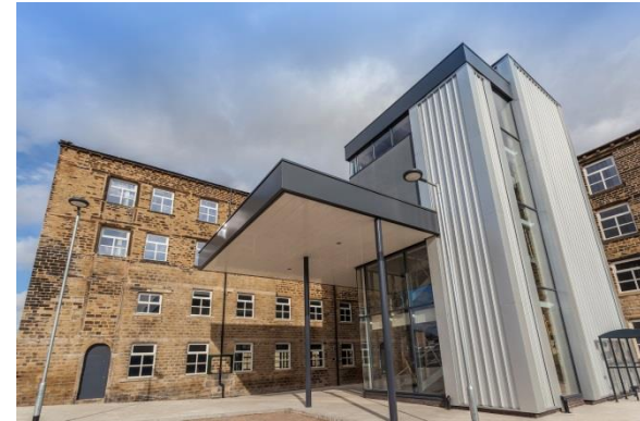
Acre Mill, Huddersfield – completed redevelopment
