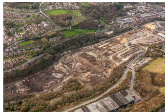
Fox Valley, Stocksbridge – 15 acre redevelopment of former steelworks
