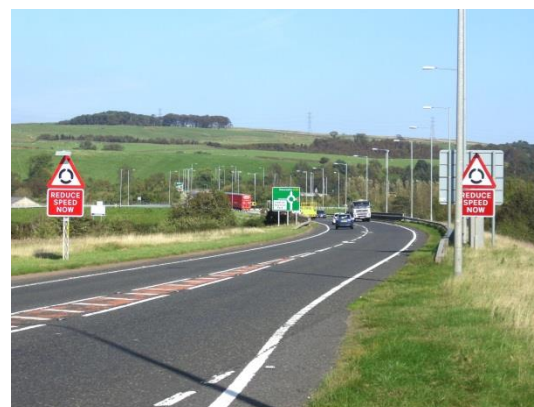
Road maintenance by Road Link (A69) Limited
