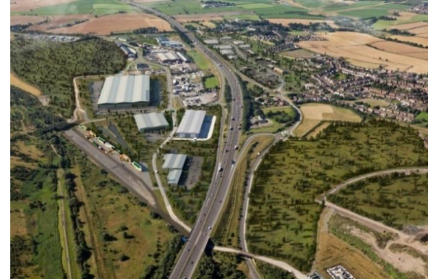
Markham Vale, Derbyshire - 200 acre development
