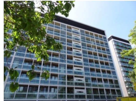
Refurbishment for Eastland Homes, Manchester
